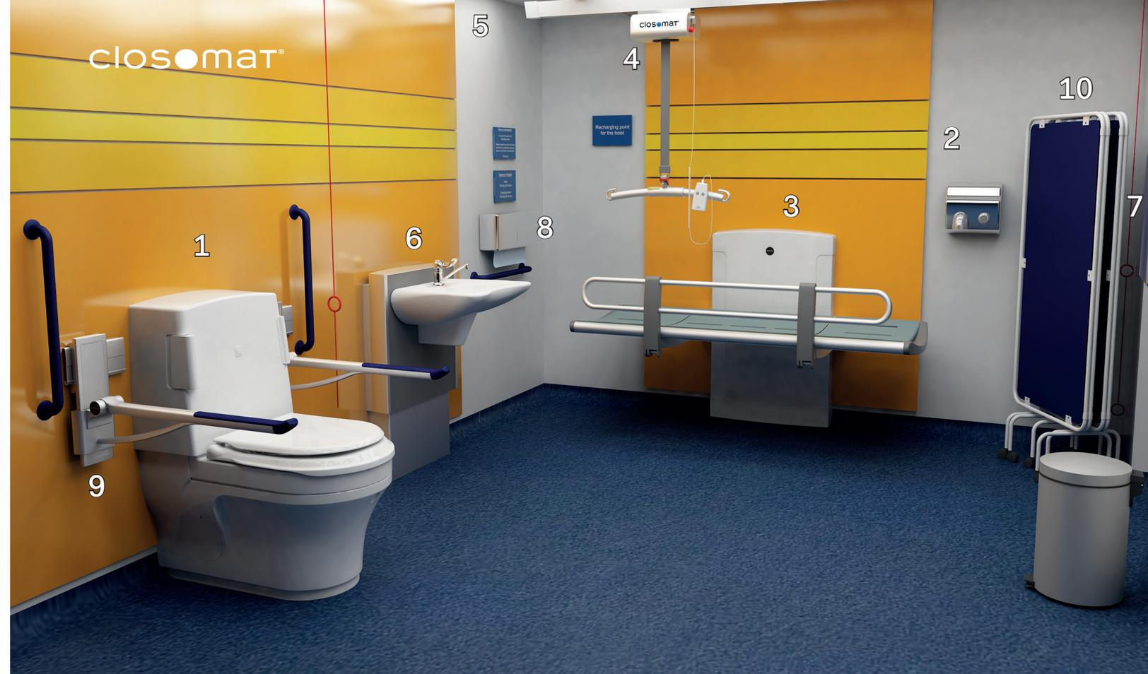
9. WC: peninsular, to allow transfer, access from either side (at least 1m from the nearest wall to the centre of the WC) NB BS8300:2018 notes that a wash & dry toilet in place of a conventional WC adds dignity and independence for users
